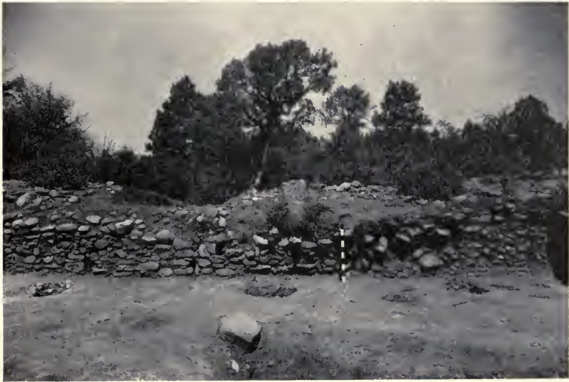
FIG. 6. West wall of Sawmill Site kiva. Meter stick for scale.
