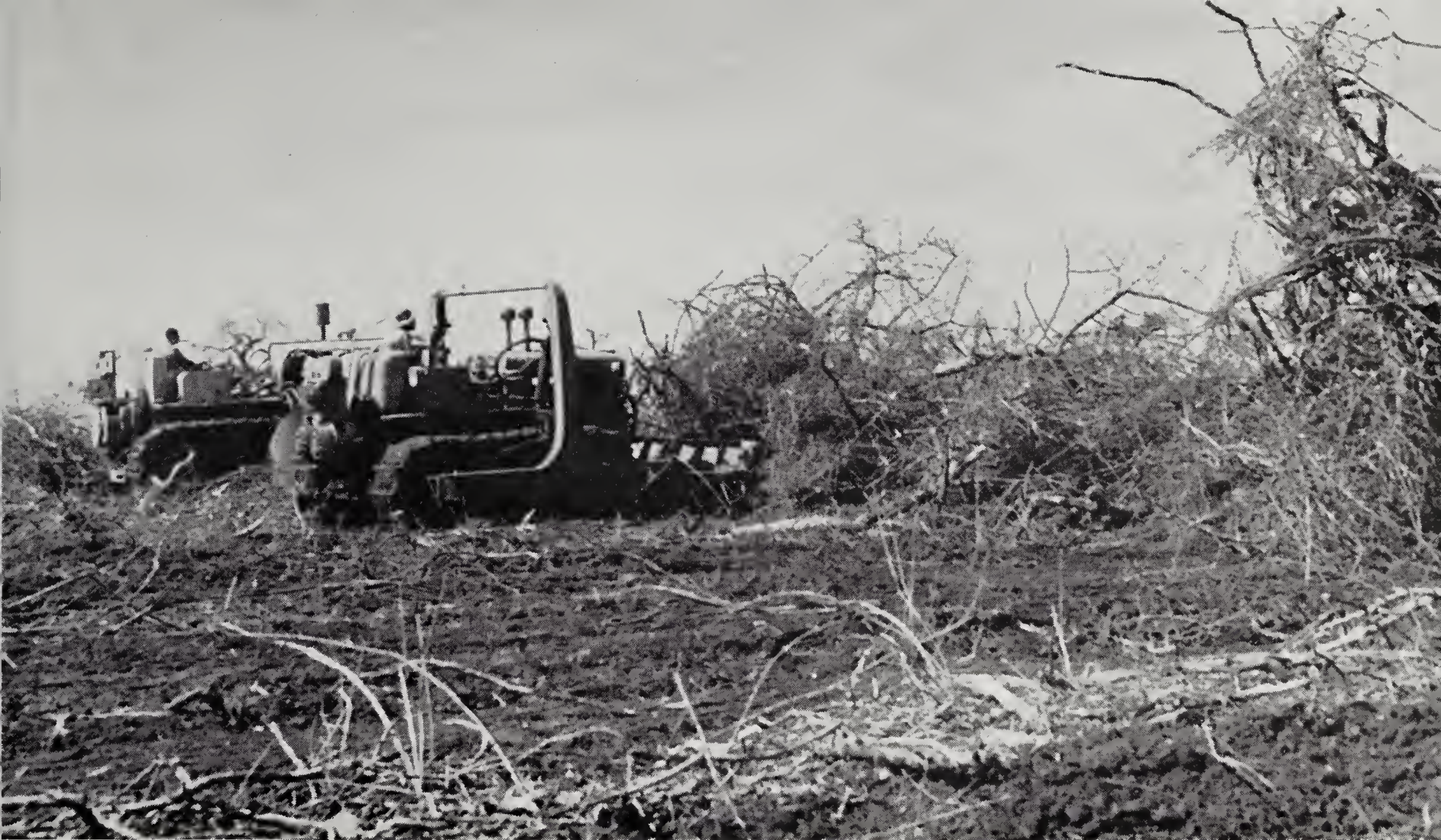
Cut scrub is bulldozed to form windbreaks
